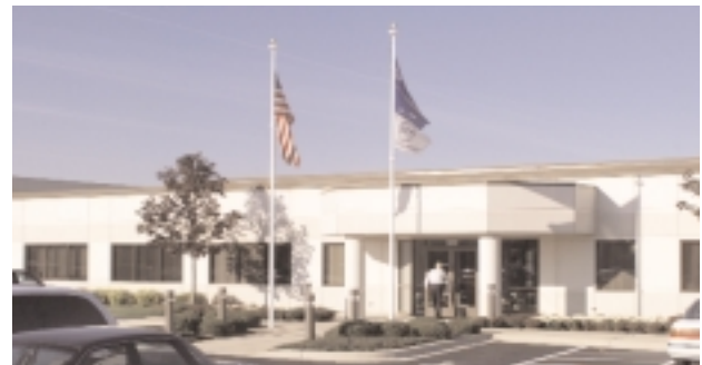
CEF Industries facilities in Addison, Illinois, near Chicago's O'Hare International Airport
